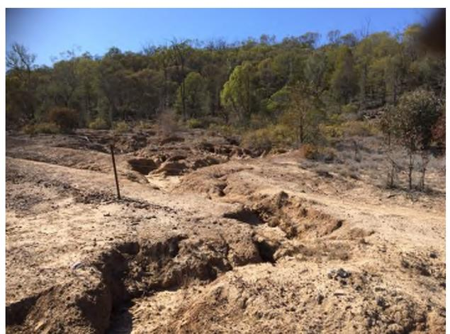
Plate 4 – Existing erosion on the south-western slopes and condition of fencing.
